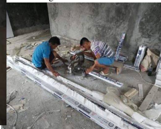
Our windows are aluminum. The two workers are sizing and cutting the window frames.
