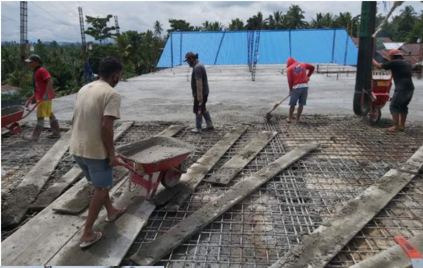
They are about 26 hours into the pour.
